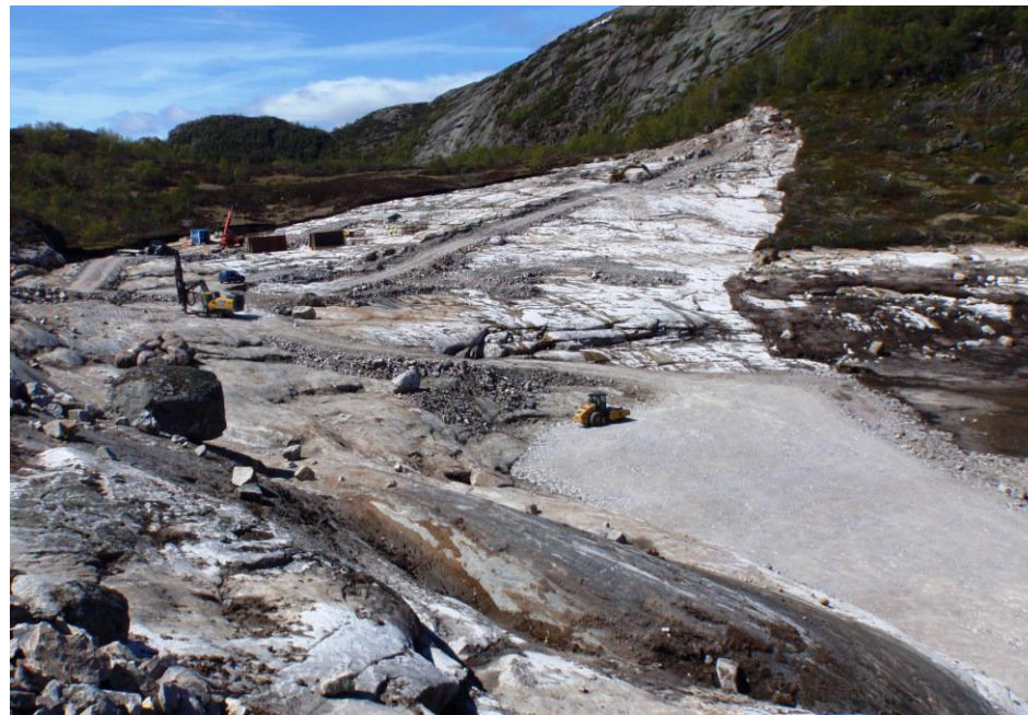
Foundation at dam HEDDERSVIKA
