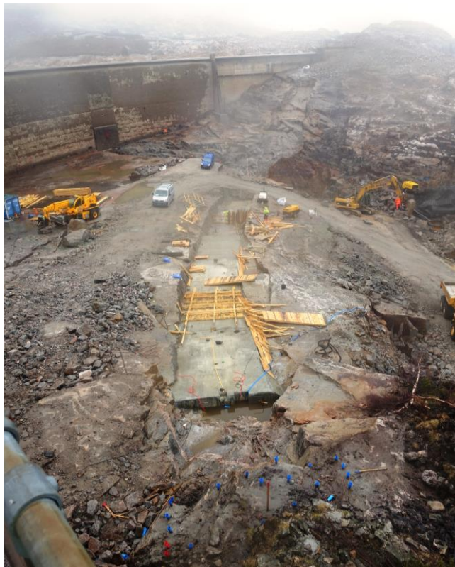
Plinth construction at new dam SKJERKEVATN
