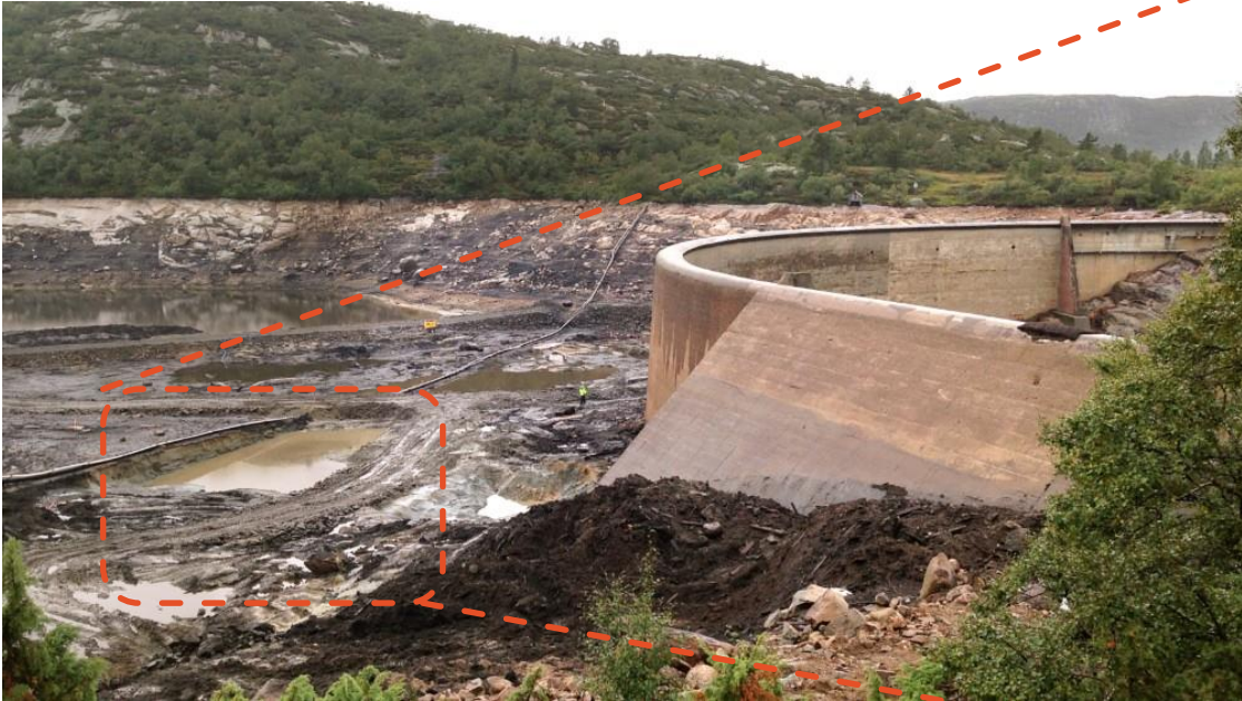
Dumping area at existing dam SKJERKEVATN
